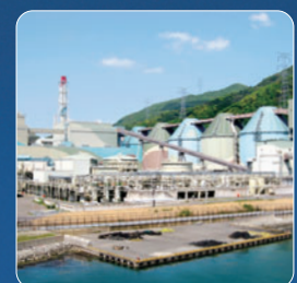
Maizuru Thermal Power Station
