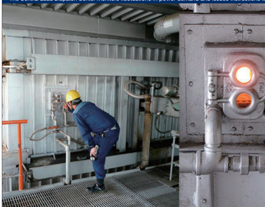
Inspection of boiler
