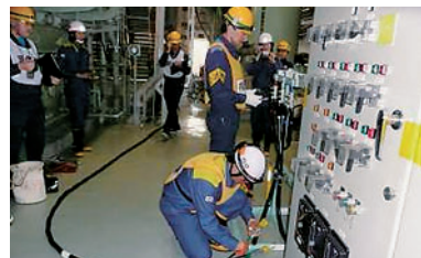
Power-supply car cable connection training
