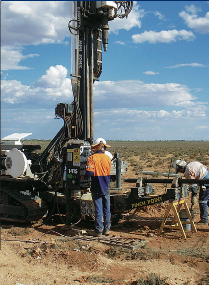
Development site of uranium mine in Australia
