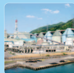
Maizuru Thermal Power Station
