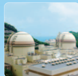
Ohi Nuclear Power Station
