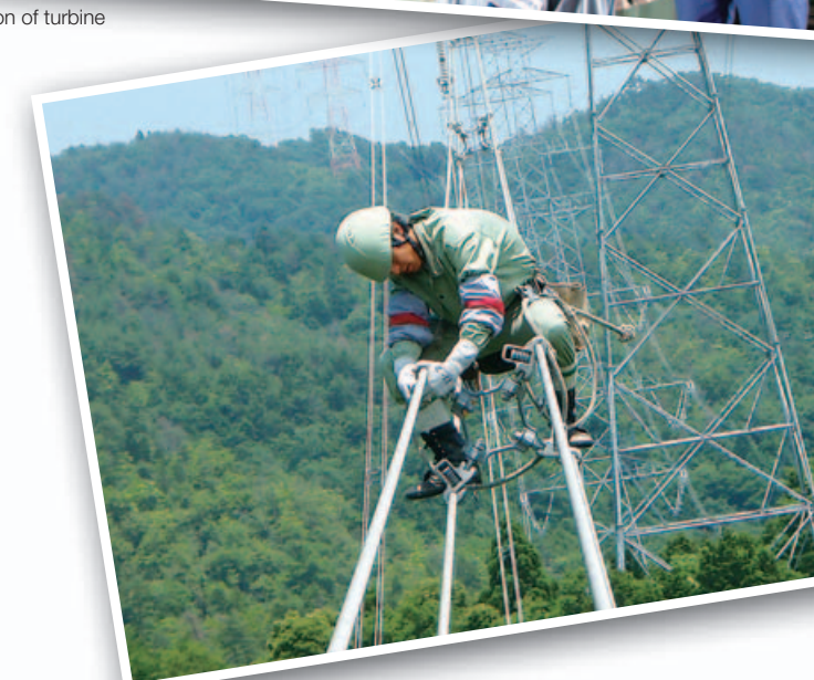
Maintenance on transmission lines
