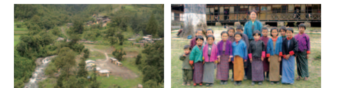
Bhutan Micro Hydro Power Project
