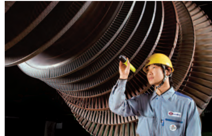
Inspecting the turbine at a power plant
