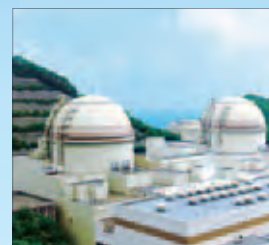
Ohi Nuclear Power Plant
