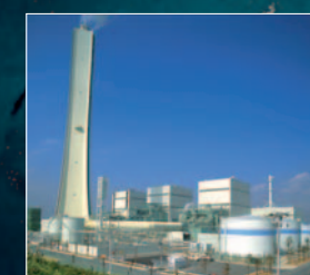
Nanko Thermal Power Plant
