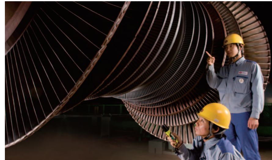
Inspecting the turbine at a power plant
