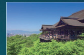
The main temple and stage of Kiyomizu Temple in Kyoto, a national treasure
