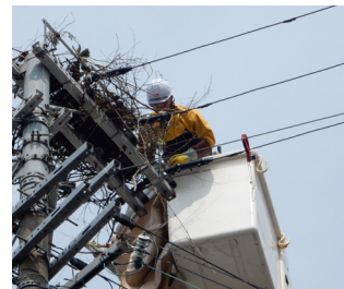
Checking the condition of utility poles
