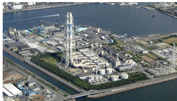
Himeji No. 1 Power Station
