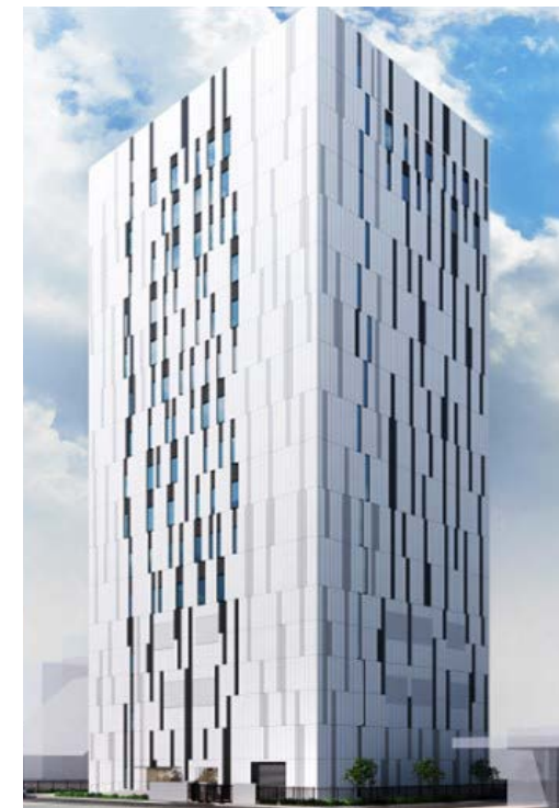
Sonezaki Data Center (OC1) Operation to start in January 2026
