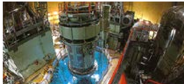
Removing the lid of a nuclear reactor pressure vessel at the Mihama Nuclear Power Station
