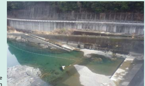
Fish passage installation
