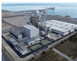
Biomass: Kanda Biomass Power Plant
