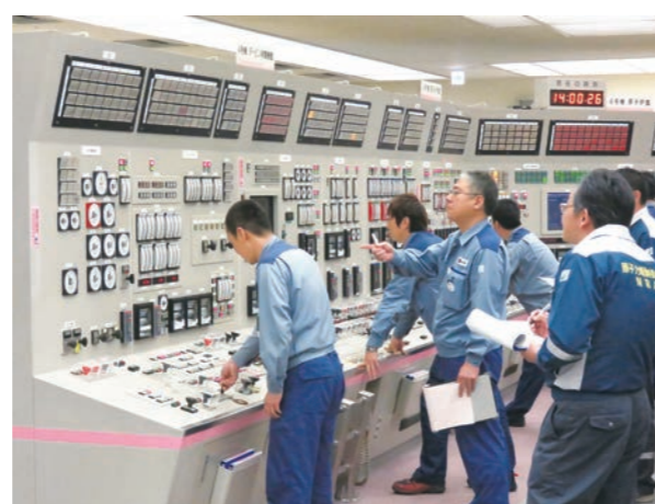
Operators connecting Takahama Power Station Unit 4 to the transmission network
