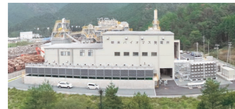
Asago Biomass Power Plant
