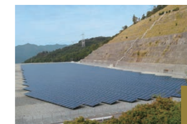
Yamazaki Solar Power Station
