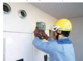
Smart meter installation work
