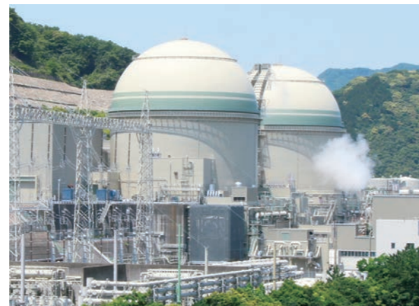
Takahama Power Station Units 3 and 4 have resumed operation
