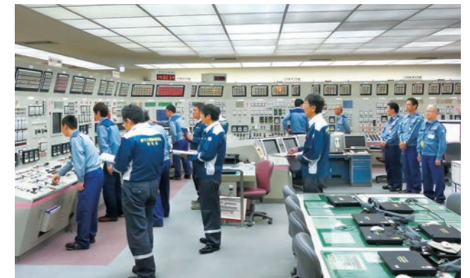
Central Control Room at the time power generation started
