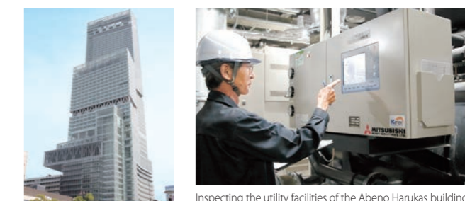
Inspecting the utility facilities of the Abeno Harukas building
