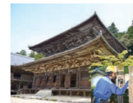
Shoshazan Engyo-ji temple electrical equipment diagnostics
