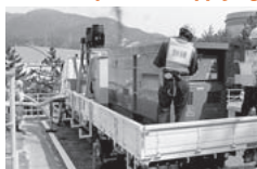
Installation of a medium-pressure pump to supply water to the steam generator
