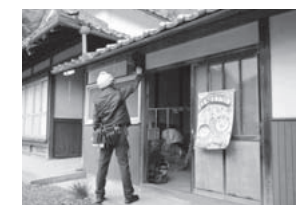
Electrical equipment inspection for housing for elderly persons
