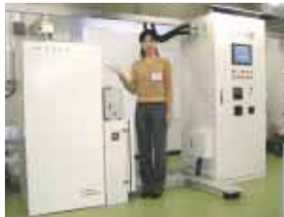
1-kW SOFC power generation system that we developed
