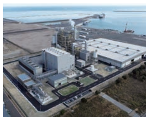
Biomass: Kanda Biomass Power Plant
