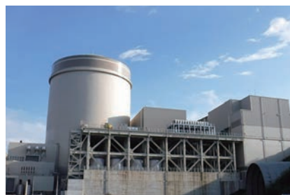
Mihama Nuclear Power Station Unit 3, back in operation
