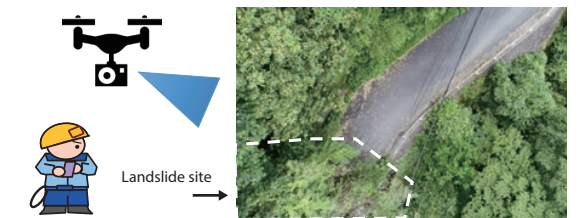
Damage investigation by aerial drone video
