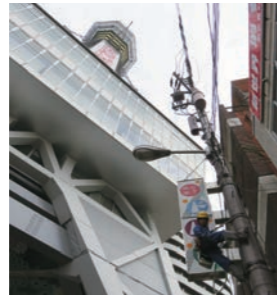
Inspecting electrical equipment at the Tsutenkaku Tower
