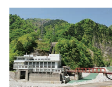
Kurobegawa No. 2 Hydropower Plant
