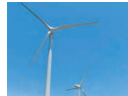
Tahara No. 4 Wind Power Station
