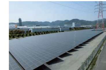
Ako Nishihama Solar Power Station
