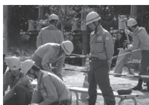
On-the-job training for repair work
