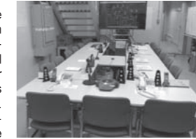
Ohi Power Station Units 1 and 2 Conference room next to the main control room (emergency response center)
