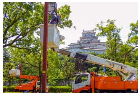
Cleaning of streetlights around Himeji Castle using aerial work platforms, Hyogo
