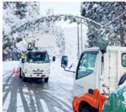
Restoration of utility poles damaged due to heavy snow
