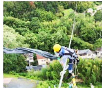
Removal of blown debris from power lines
