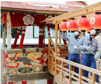
Electrical wiring inspection for Gion Festival floats, Kyoto
