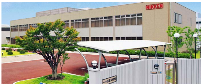
Nikken Kosakusho Works and their solar panels
