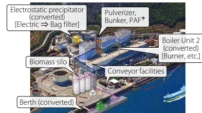
* A ventilator that feeds pulverized fuel to burners
