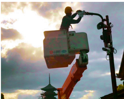
Cleaning of lighting equipment at Toji Temple, Kyoto
