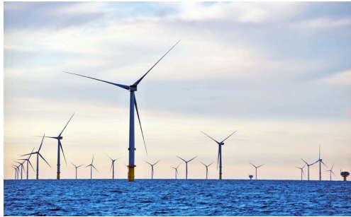
Triton Knoll Offshore Wind Power Project in the UK
