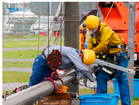
Restoration work training in preparation for a disaster
