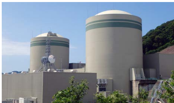
Takahama Nuclear Power Station Units 1 and 2 containment vessel upper shield installation work
