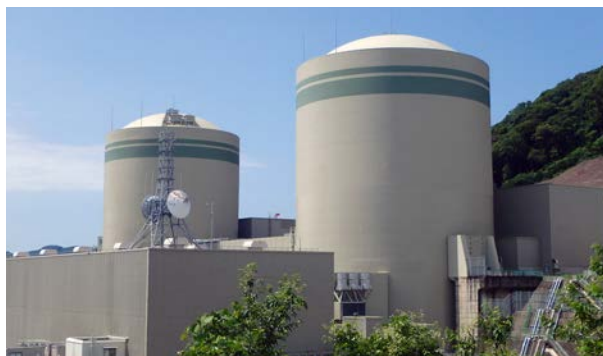
Takahama Nuclear Power Station Units 1 and 2 containment vessel upper shield installation work
