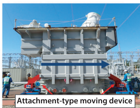
New construction method using an attachment-type moving device
