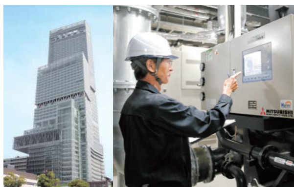
Inspecting the utility facilities of the Abeno Harukas building
