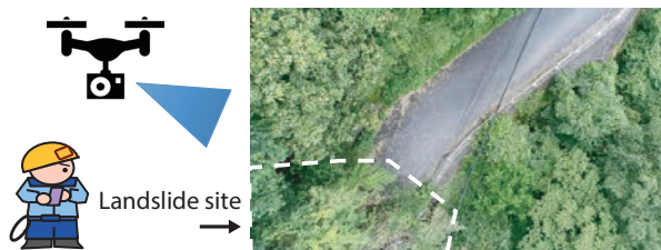
Damage investigation by aerial drone video
