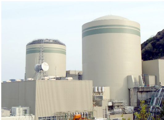
Takahama Nuclear Power Station Units 1 and 2 containment vessel upper shield installation work
