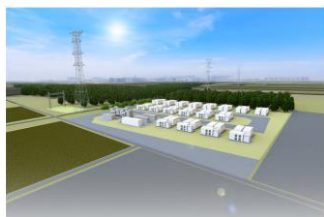
Mito Energy Storage Plant
