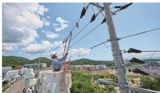
Distribution Line Inspection
