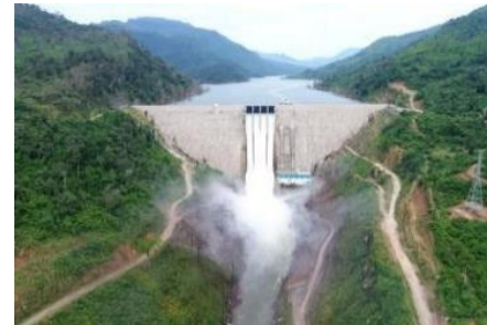
Nam Ngiep 1 Hydropower Project
