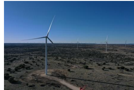
Aviator Onshore Wind Farm Project
