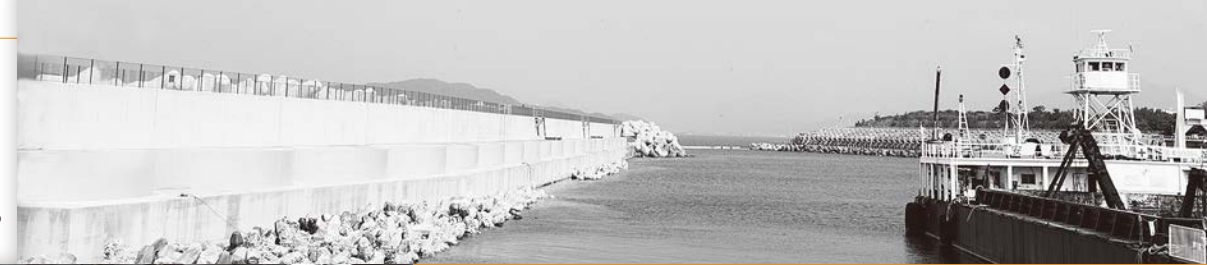
▶海拔5mから8mに嵩上げた防波堤
