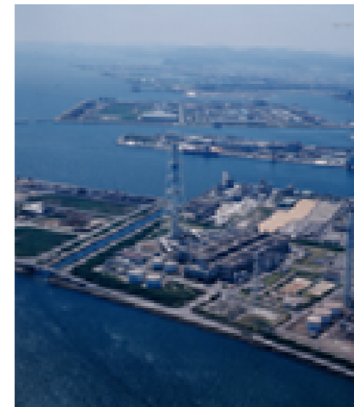
Himeji No.1 Thermal Power Plant (1,442 MW)
