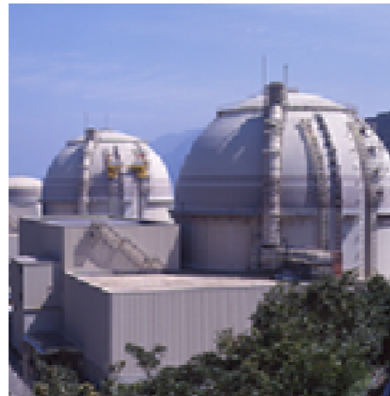
Ohi Nuclear Power Plant (4,710 MW)
