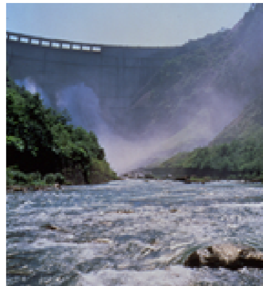
Kurobegawa No.4 Hydro Power Plant (335 MW)
