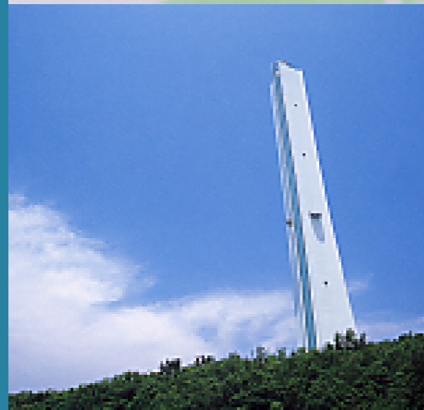
Nanko Thermal Plant
