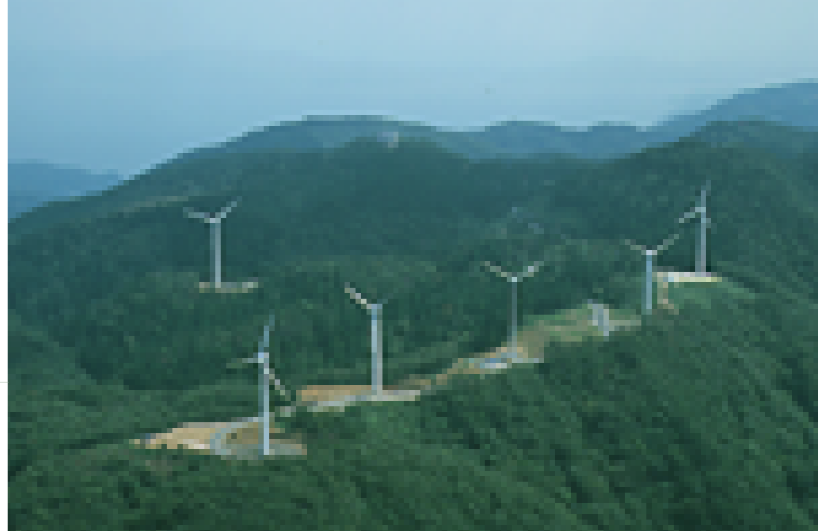
Wind-power generation equipment supported by the Kansai Green Power Fund (Taiko-yama, Kyoto)
