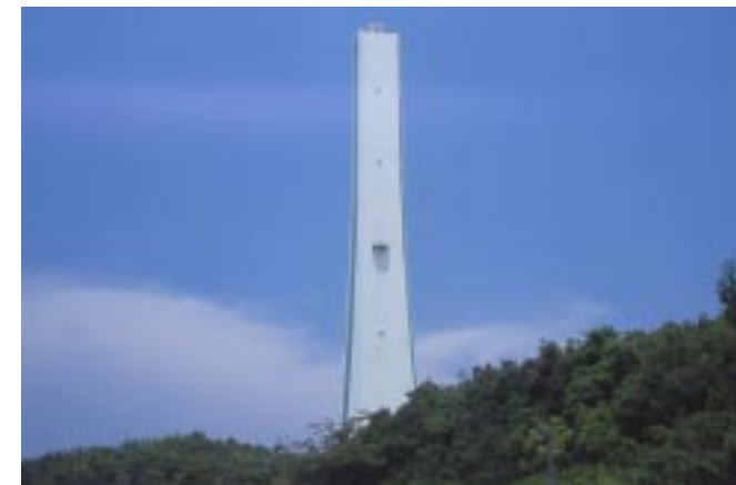
Nanko Thermal Power Plant
