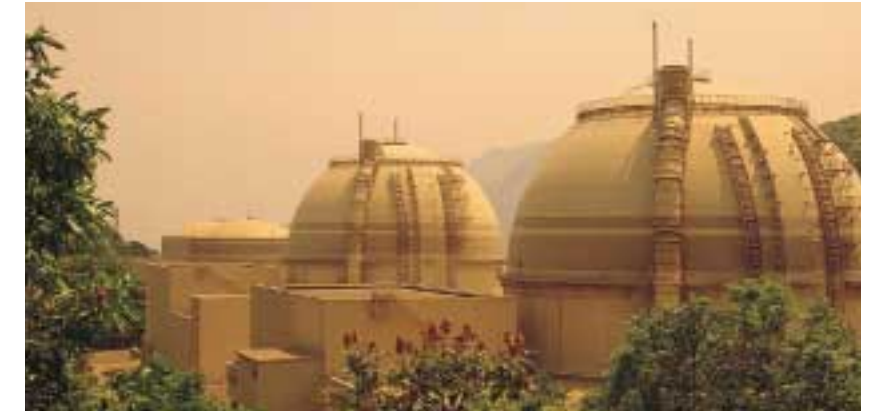
Ohi Nuclear Power Plant. The Ohi Plant, boasting an output of 4,710 MW, is Kansai EP's largest nuclear power station.
