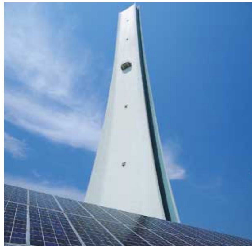
Solar panels installed at Nanko Fossil Fuel Power Plant.
