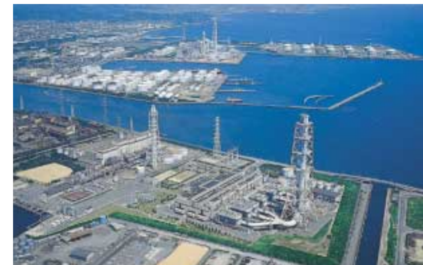
Himeji No.1 Combined Cycle Power Plant, newly certified as ISO14001 compliant.
