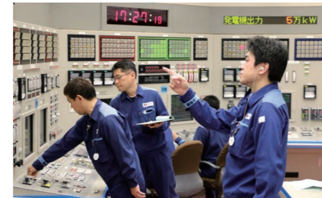
Connecting Ohi Power Station Unit 3 to the transmission network
