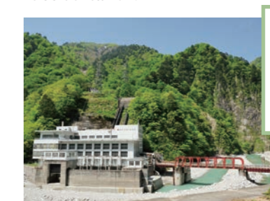
Kurobegawa No. 2 Hydropower Plant
