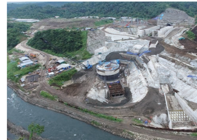
Power plants area overview
