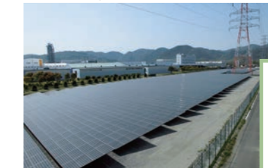
Ako Nishihama Solar Power Station
