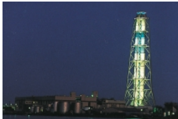
Himeji No. 1 Power Station
