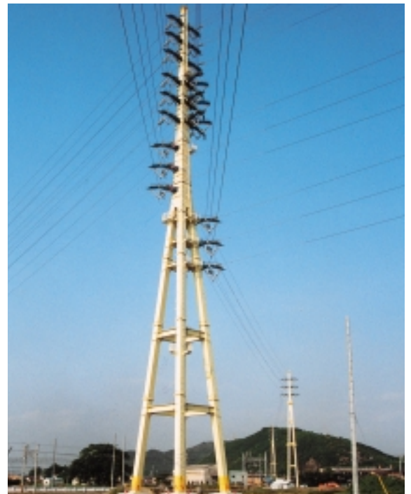
The electric transmission tower of the Himeji Power Station (fossil fuel)
