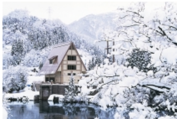
Sakaigawa Power Station
