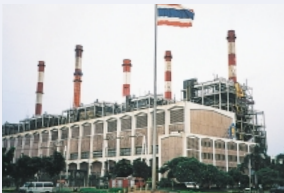
South Bangkok Power Station
