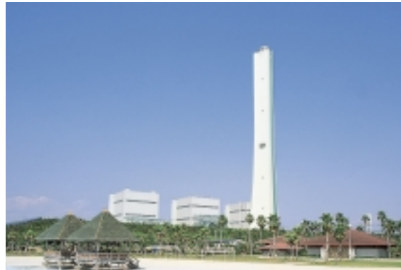
Nanko Power Station
