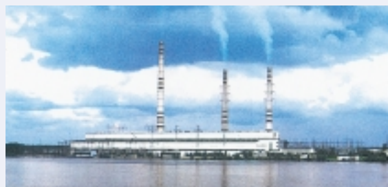
Konakovo Thermal Power Station (Moscow)
