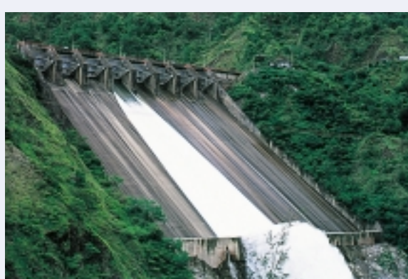
Ambuklao Hydro Electric Plant (Benguet Province, Luzon Island)
