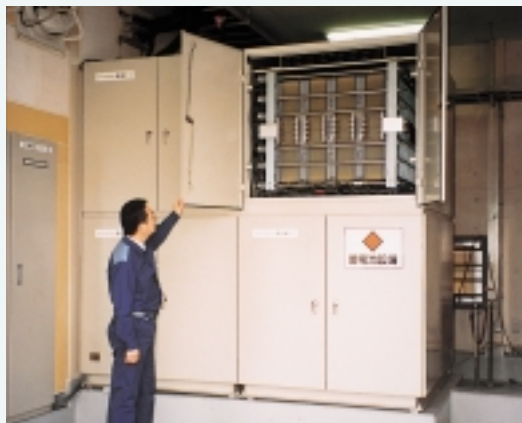
Redox flow batteries
