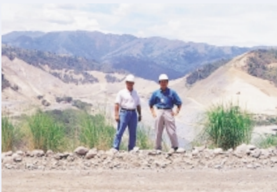
Construction site for San Roque Project
