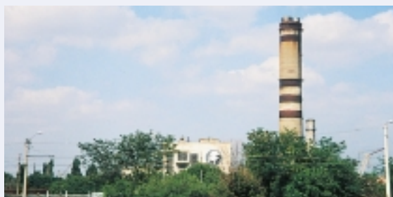
Symferopoloskaya Thermal Power Station (Crimea)
