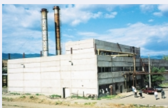
District Heating Plant in Tbilisi, Georgia
