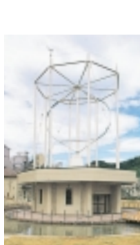
Darrius wind turbine power generator
