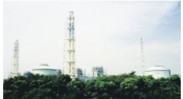
Ecological greening (Himeji No. 2 Power Station)
