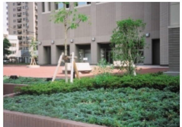
Green space in open area around city substation (Uehonmachi Substation)
