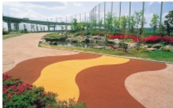
Water-permeable pavement from insulator scraps (Amagasaki Techno-land)
