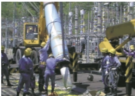
Removal of bushing from transformer (Nishi-Harima Transformer Substation)
