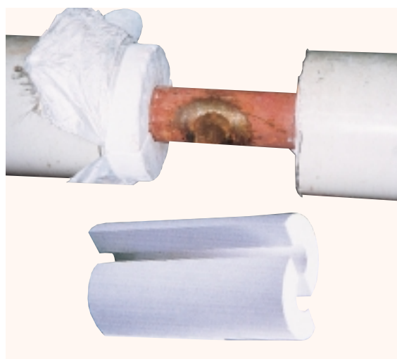
Insulation material for piping at power station
