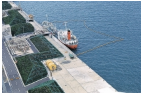
Oil fence at unloading dock
