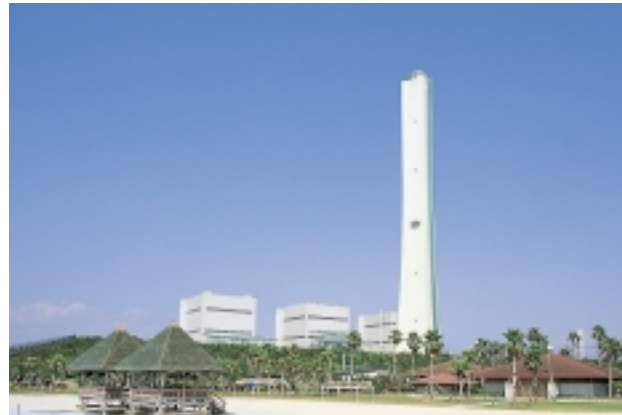
Nanko Power Station
