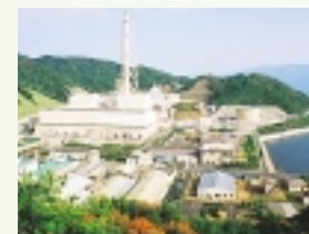
Miyazu Energy Research Center
