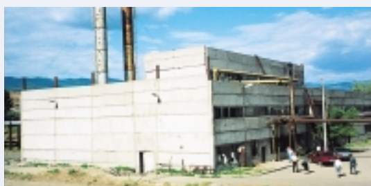
District Heating Plant in Tbilisi, Georgia
