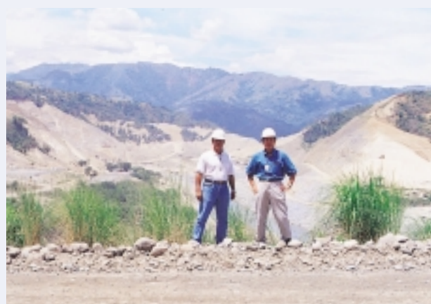
Construction site for San Roque Project
