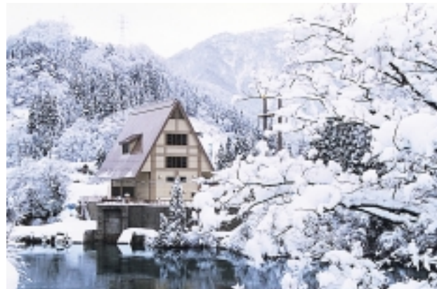
Sakaigawa Power Station
