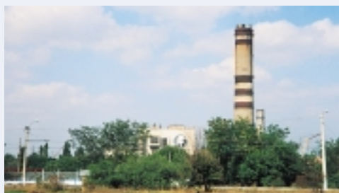
Symferopolskaya Thermal Power Station (Crimea)
