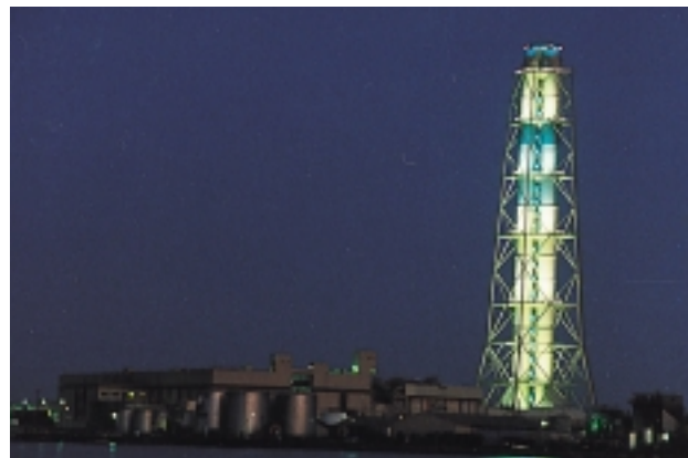
Himeji No. 1 Power Station
