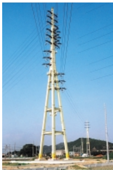
The electric transmission tower of the Himeji Power Station (fossil fuel)
