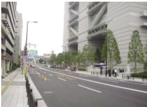
The area around Osaka International Conference Center (underground power lines)
