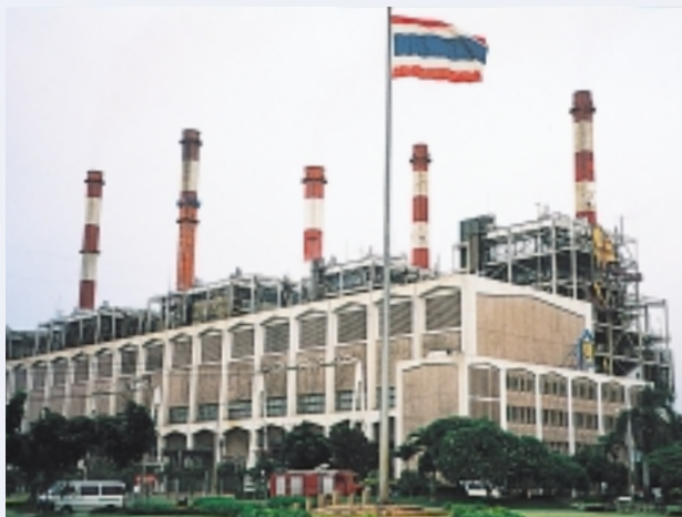
South Bangkok Power Station
