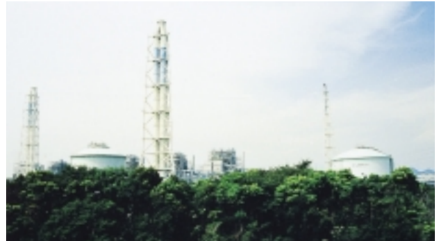
Green zone at the Himeji No. 2 Power Station
