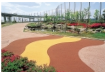
Water-permeable pavement from insulator scraps (Amagasaki Techno-land)
