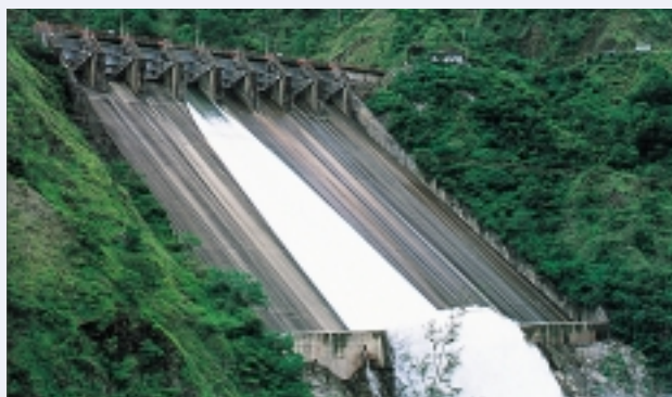
Ambuklao Hydro Electric Plant (Benguet Province, Luzon Island)
