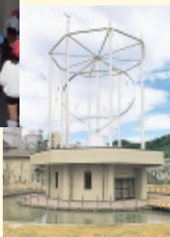
Darrieus wind turbine power generator
