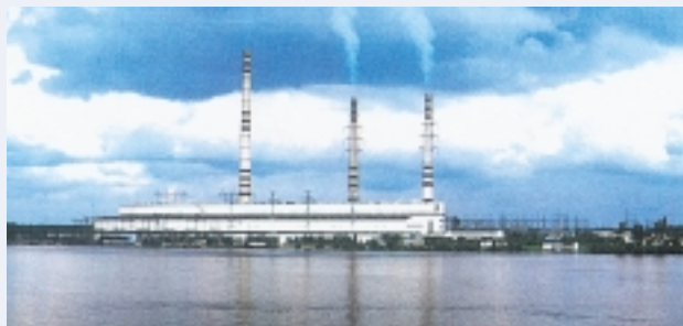
Konakovo Thermal Power Station (Moscow)
