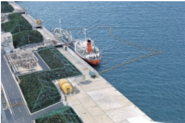
Oil fence at unloading dock
