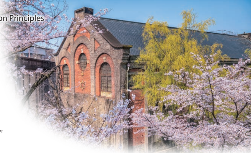
Keage Power Station, open to the public from March 2018
