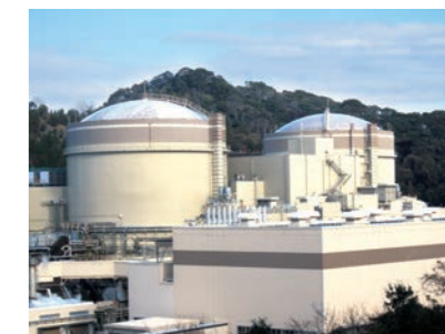
Ohi Nuclear Power Station Units 1 & 2
