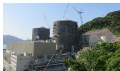
Takahama Nuclear Power Station Units 1 and 2 containment vessel upper shield installation work
