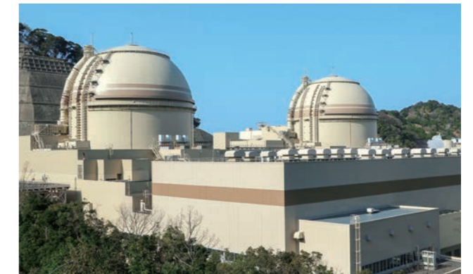
Ohi Nuclear Power Station Units 3 & 4
