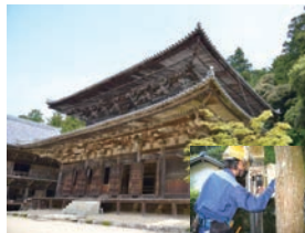
Shoshazan Engyo-ji temple electrical equipment diagnostics
