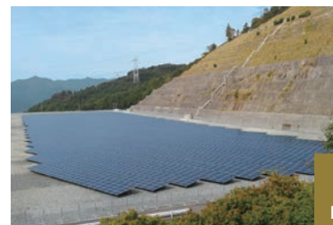
Yamazaki Solar Power Station
