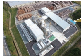
Asago Biomass Power Plant
