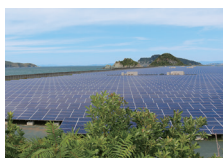
Arida Solar Power Station
