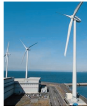
Tahara No. 4 Wind Power Station
