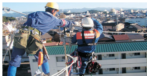
Rescue training on a steel tower
