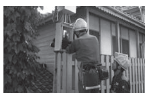
Inspecting electrical equipment at the Moegi House of the Kitano Foreign Residences in Kobe-shi, Hyogo
