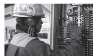
Inspecting electrical equipment at the Kagiya Museum, a landmark architectural site in Hirakata-shi, Osaka
