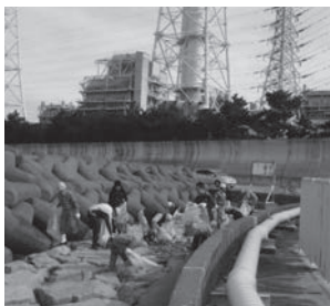
Cleanup around the Kainan Power Station in Kainan-shi, Wakayama
