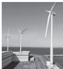
Tahara No. 4 Wind Power Station
