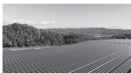
Keihanna Solar Power Station
