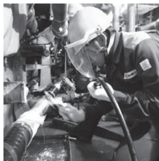
Expert cable jointer connecting cables
