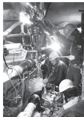
Expert cable jointer connecting cables
