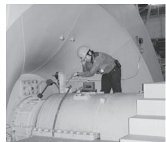
Routine inspection using a stethoscope probe
