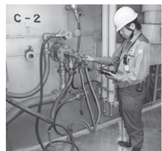
Inspection around a boiler
