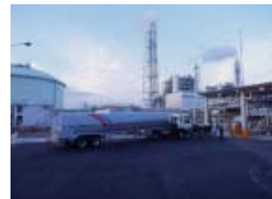
Gas shipment by tanker truck (Himeji Storage Depot)
