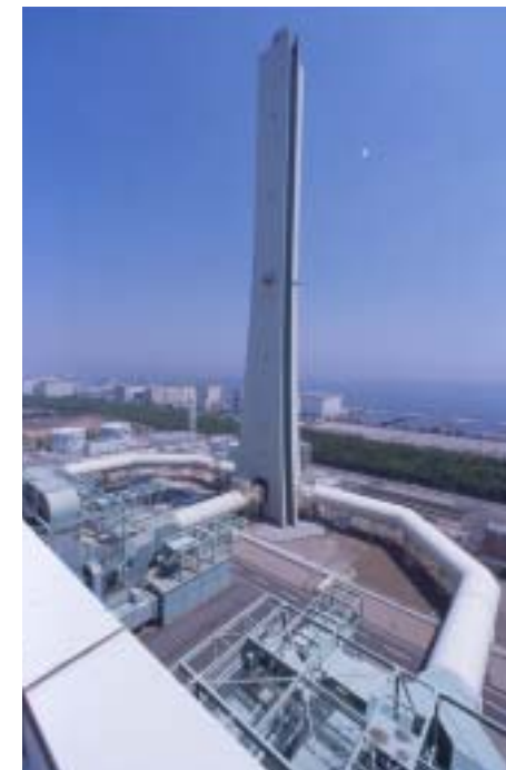
Nanko Thermal Power Plant
