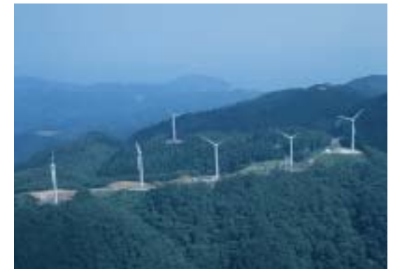
Wind-power generation equipment supported by Kansai Green Power Fund (Taiko-yama, Kyoto)
