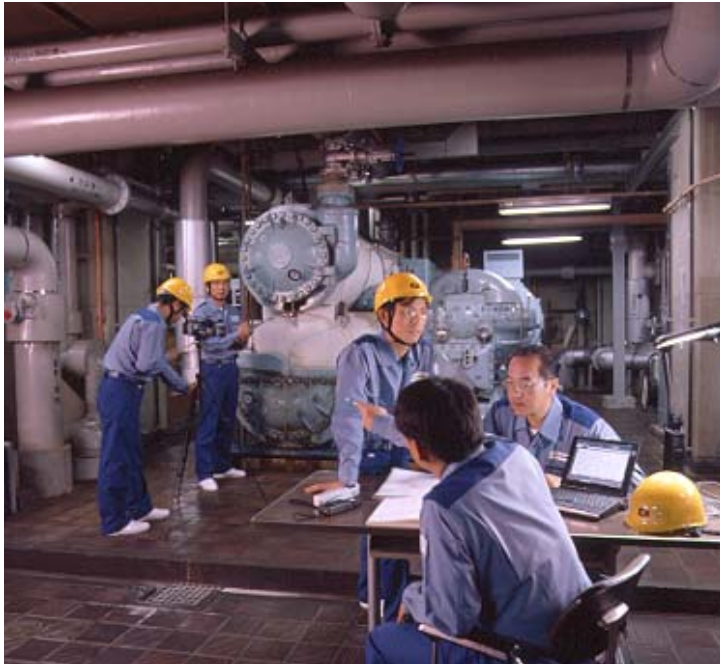
Energy equipment diagnosis
